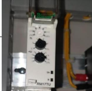
**Gambar 3.** Knob settingan *relay phase failure*
