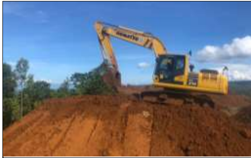
Gambar 2. Proses Penimbunan
