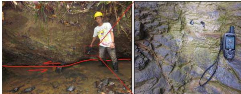
Figure 3. The Longsatu Horizontal Fault, visible fault plane, drag fold, slickenside and fractures filled by iron oxide minerals.
