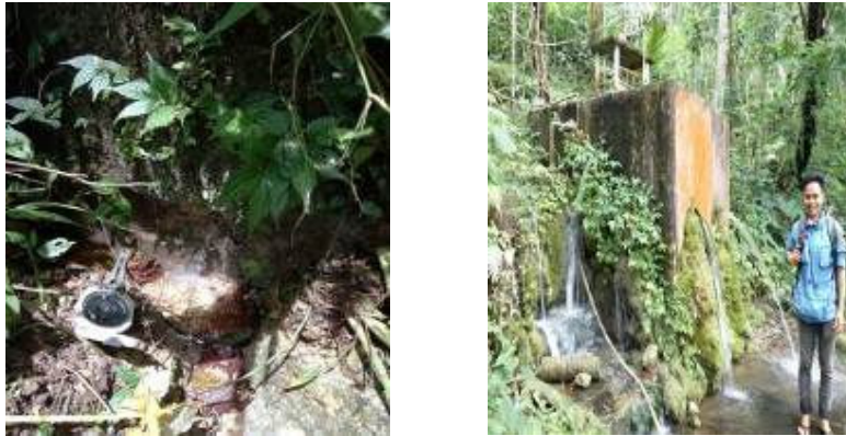
Figure 12. One of the springs (left); Water tub was built to accommodate the entire outflow of water made by residents (right).
