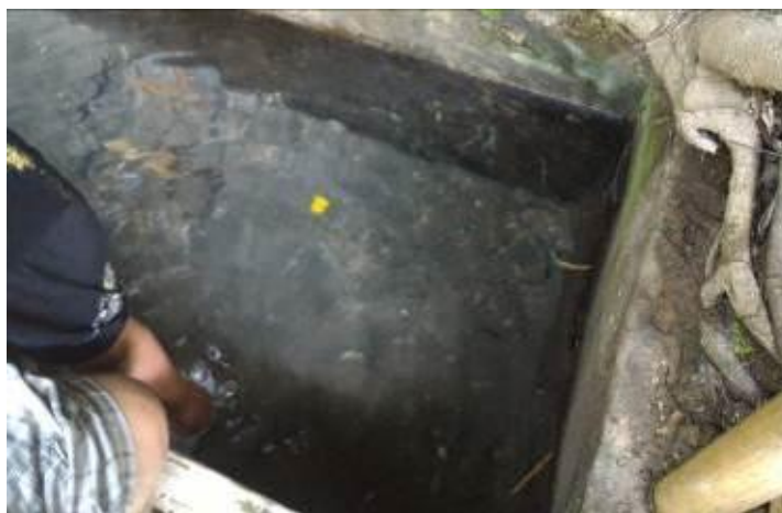
Figure 5. Dukuh spring which be constructed by concrete.
